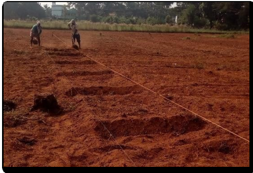
Plate 2. Initial land preparation
