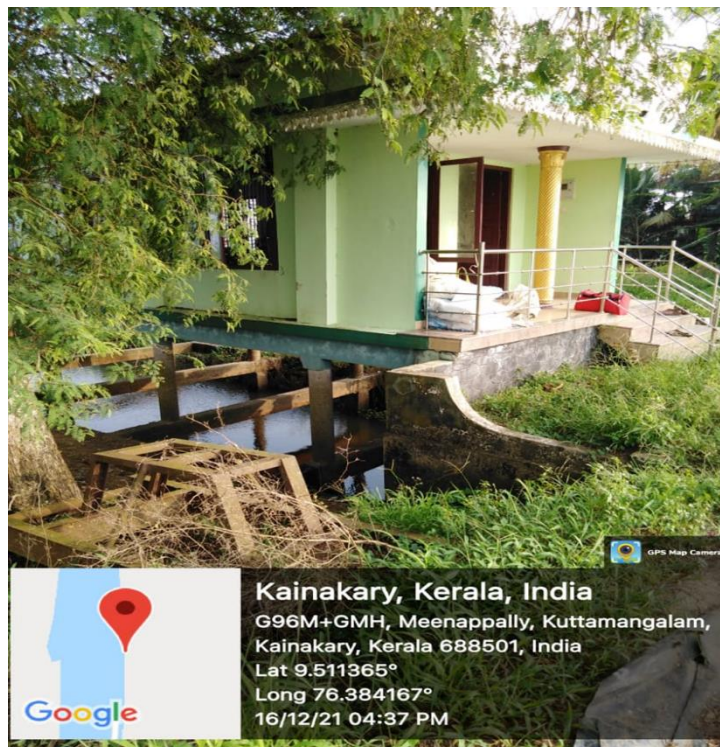
Plate 8. Houses built on cement poles in Kainakari
