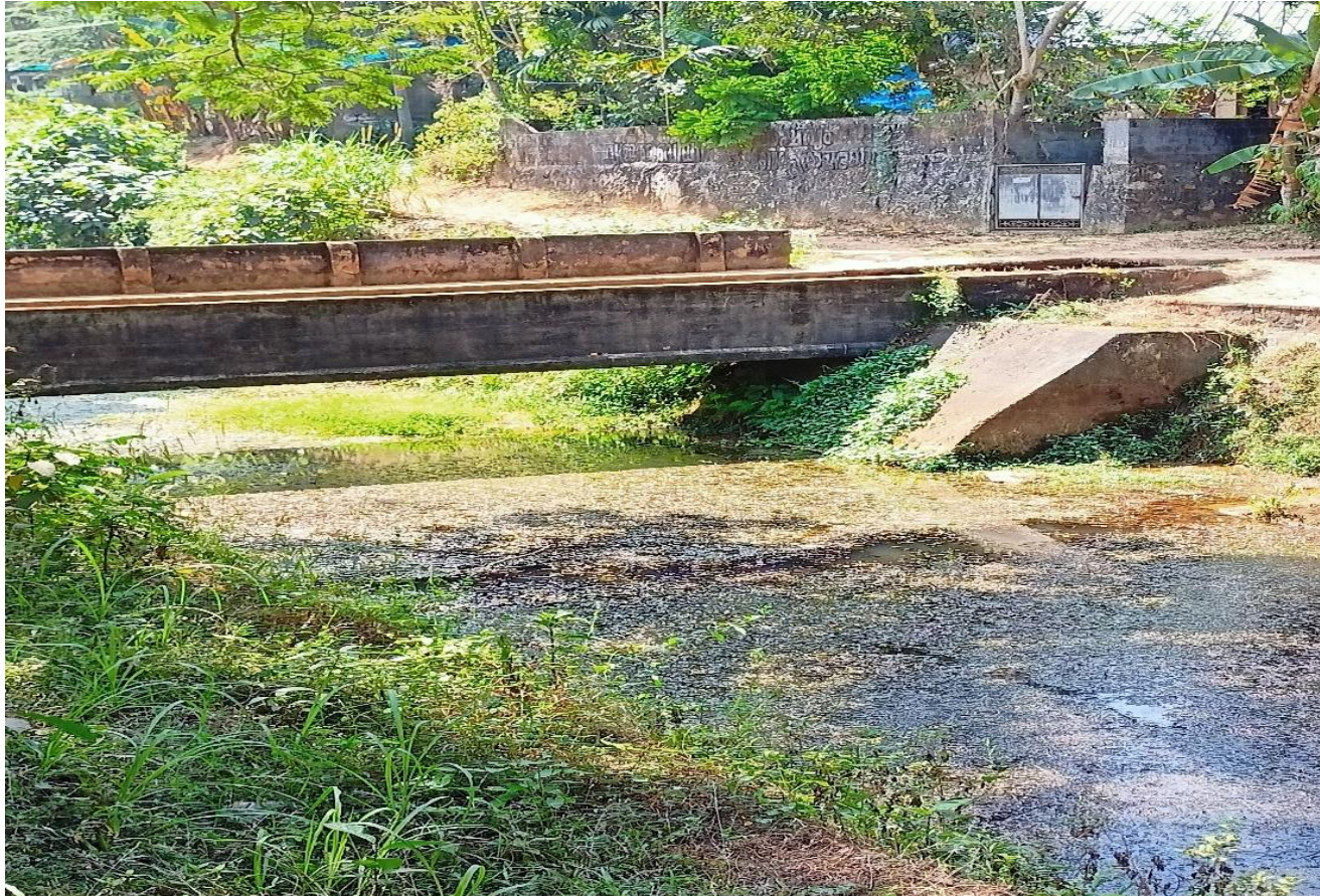
Plate 4. Siltation in Neyyar Irrigation Project canal
