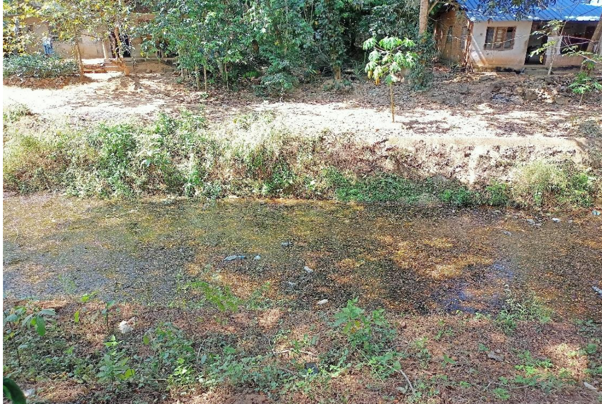
Plate 5. Poorly maintained canal of Neyyar Irrigation Project
