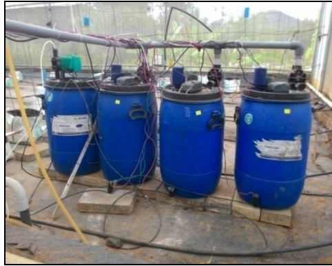
Plate 3.10 Fertilizer tank along with mixing tank and FIP arrangement
