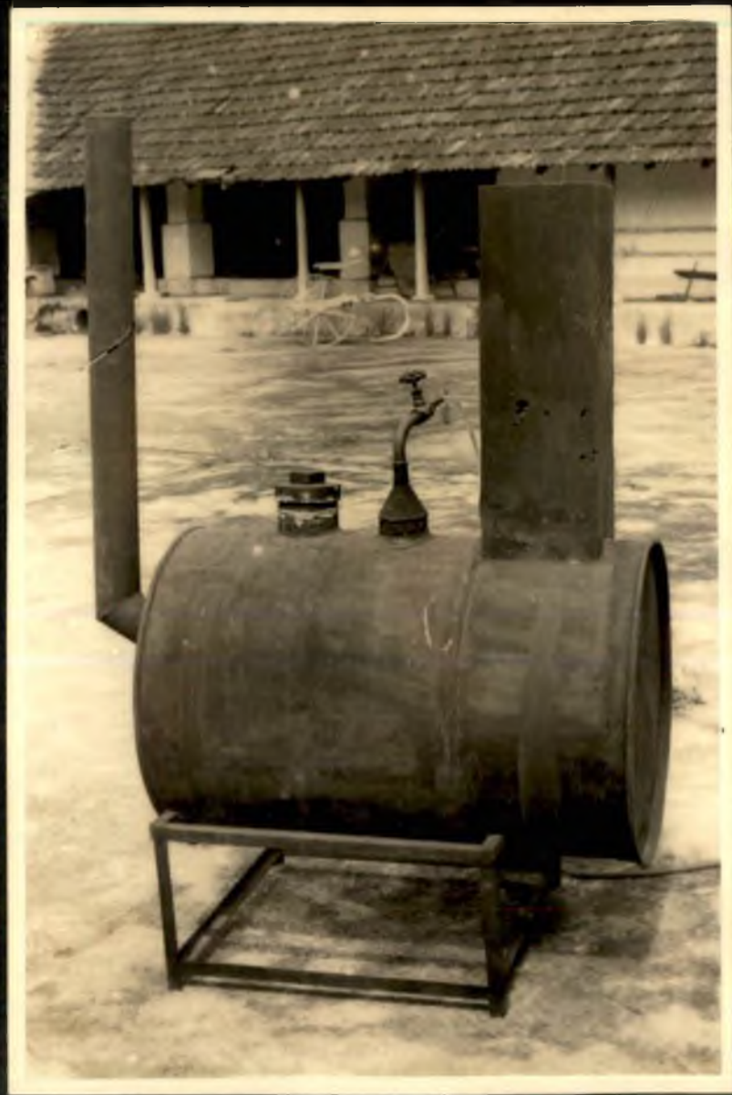
Plate III Pilot plant Horizontal K.A.U. model
