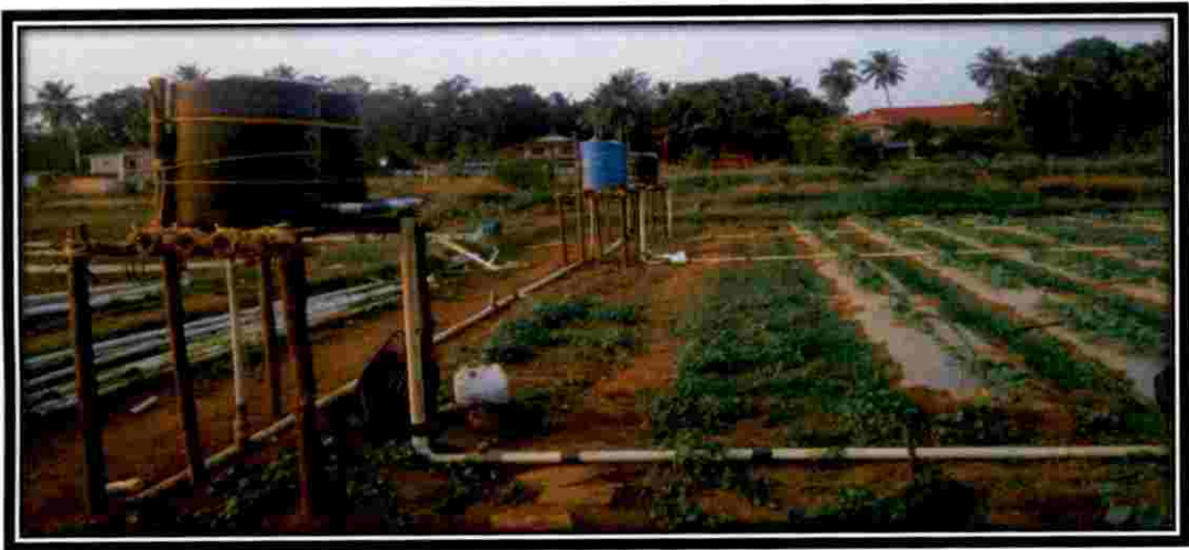
Plate 2 (a). View of experimental field after installation of drip system
