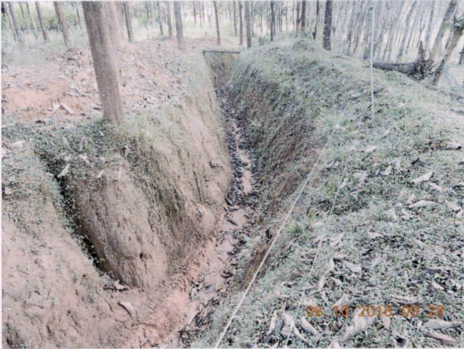
Plate 44. Elephant Proof Trench at Kallumukku, Sulthan Bathery
