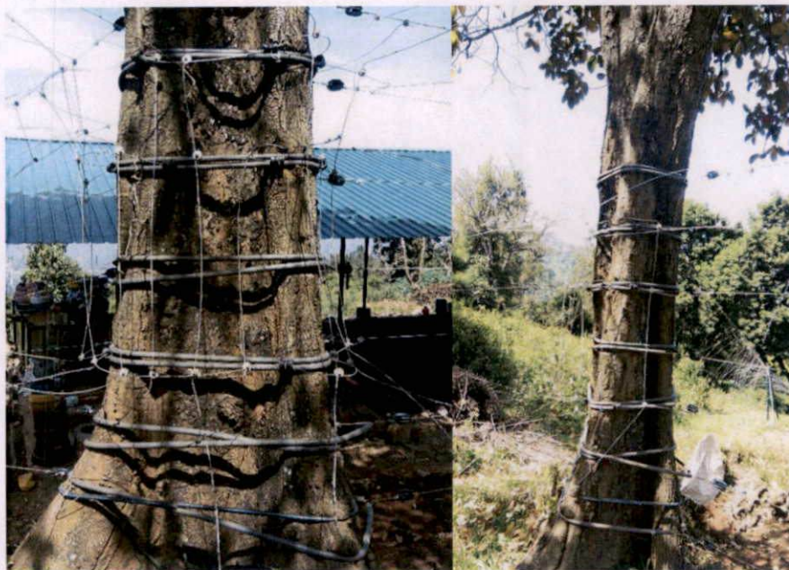
Plate 55. Electric fence to protect the dump yard with tree as support at Gudalur dump yard
