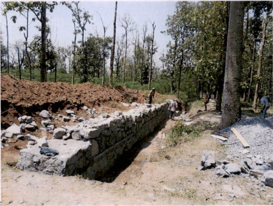
Plate 49. Elephant-proof Wall under construction at Tholpetty
