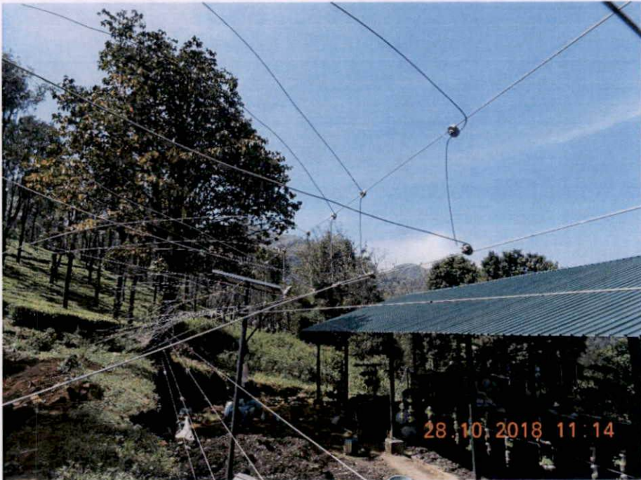
Plate 52. Tentacle fence established to prevent wild animals from entering the dump yard
