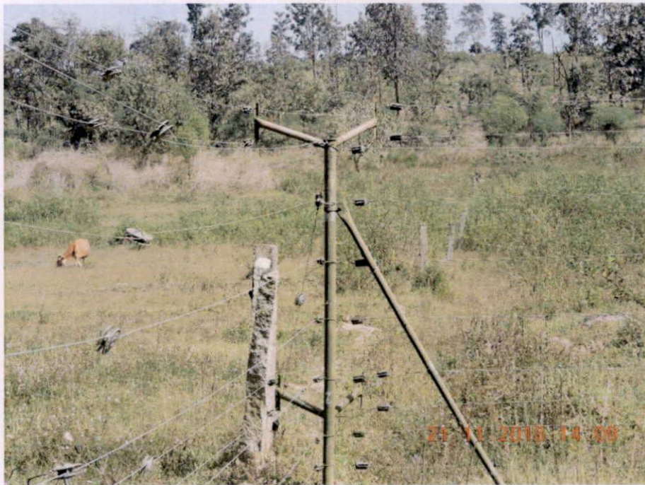
Plate 33. Well maintained private electric fence at Kallumukku, Sulthan Bathery
