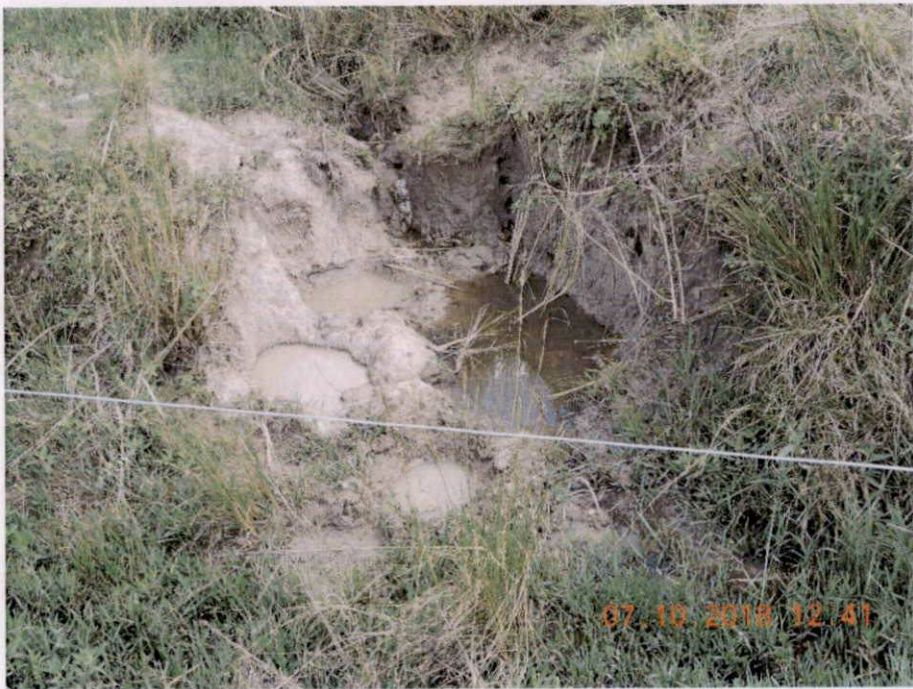
Plate 39. Elephant-proof Trench damaged by elephant at Golur, Muthanga
