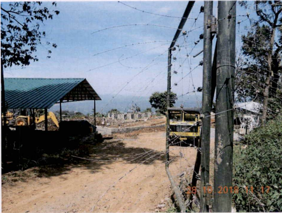
Plate 53. Gate with tentacle fence at Gudalur dump yard
