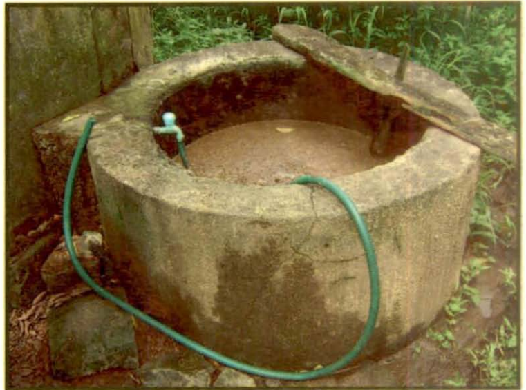
Plate 8. Inlet of biogas unit
