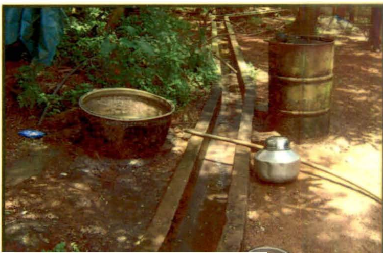
Plate 3. Separate urine channel
