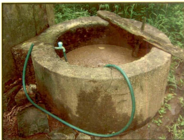
Plate 8. Inlet of biogas unit
