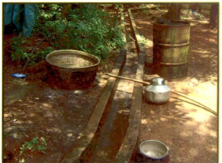
Plate 3. Separate urine channel
