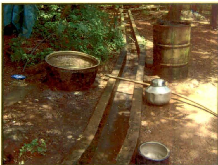
Plate 3. Separate urine channel
