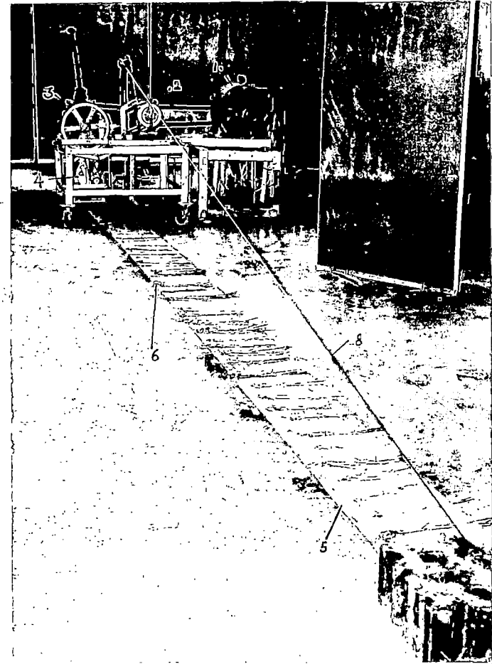
(b) View from conveyor side
