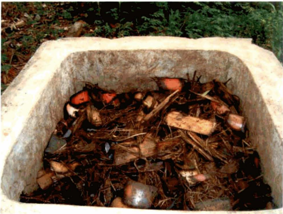
(B) Tank Overview
