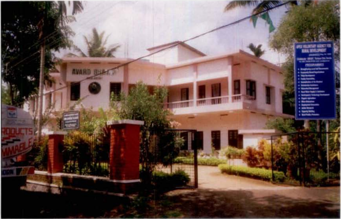
Plate 5. The main building of AVARD at Chalakudy
