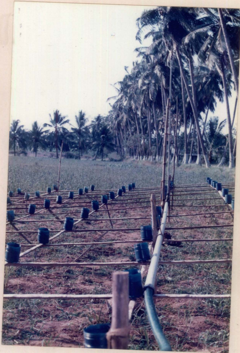
Plate 3 PVC pipe attached to the riser pipe
