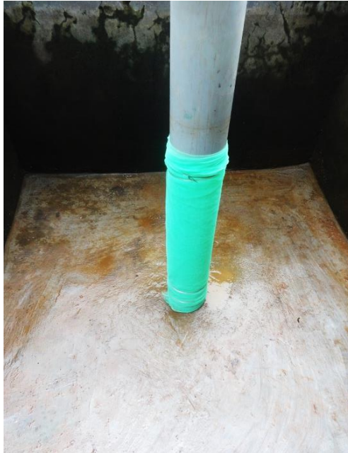
Plate 3.7 Pipe wrapped with nylon net
