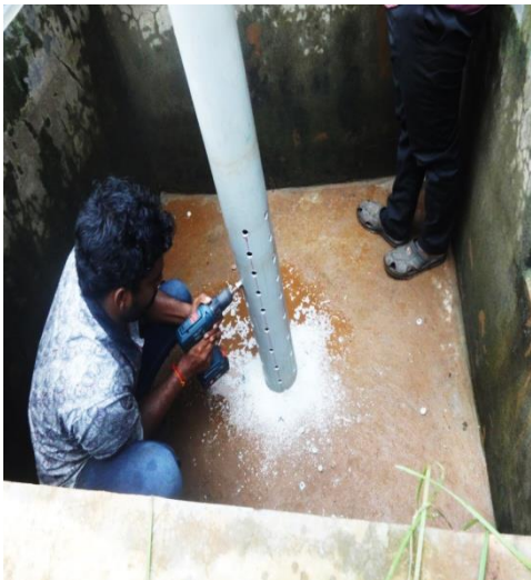
Plate 3.6 (A) Drilling holes in the pipe Plate 3.6 (B) View of holes made in the pipe
